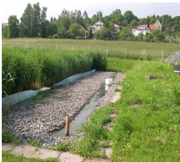
Figure 3.6 Ondřejov HF wetland: HF bed with vegetation and inlet distribution zone. Photo courtesy of Jan Vymazal.
